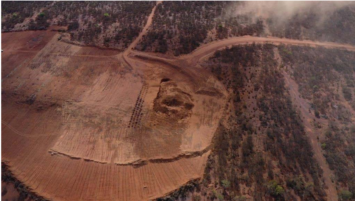
Figure 2: Production Drill Blasting Commenced
