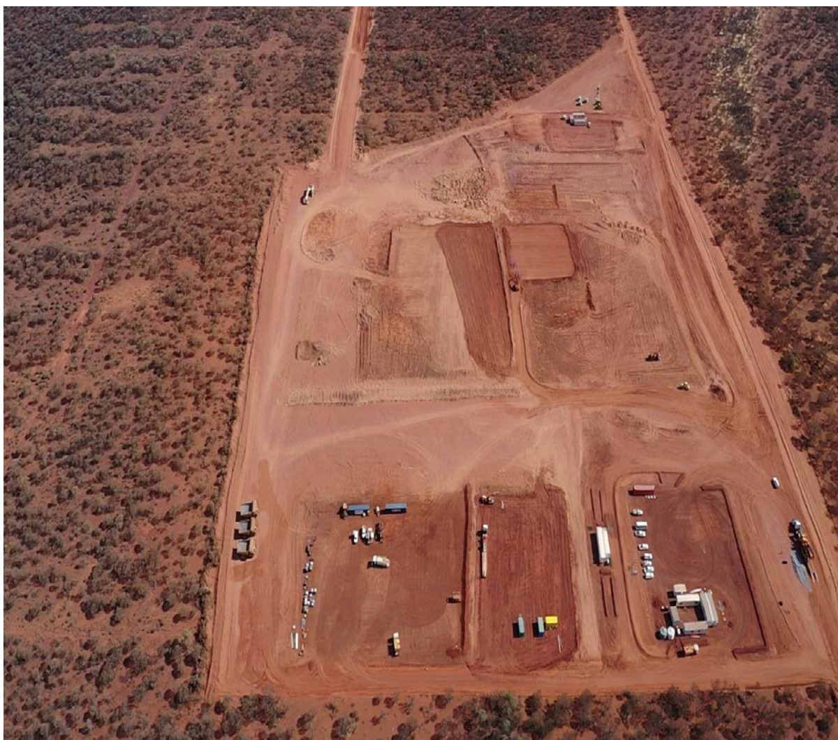
Figure 1: C4 Iron Deposit Site Operations including ROM Pads and other facilities
