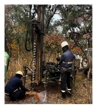
Figure 3: Auger drilling underway at Diobi, December 2023
