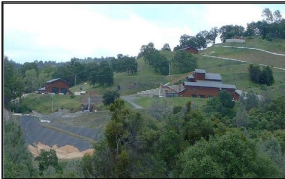
Waste Rock Pad Bottom Left
