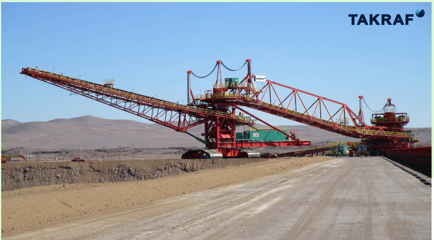
Image 3 TAKRAF Conveyor Stacking System
