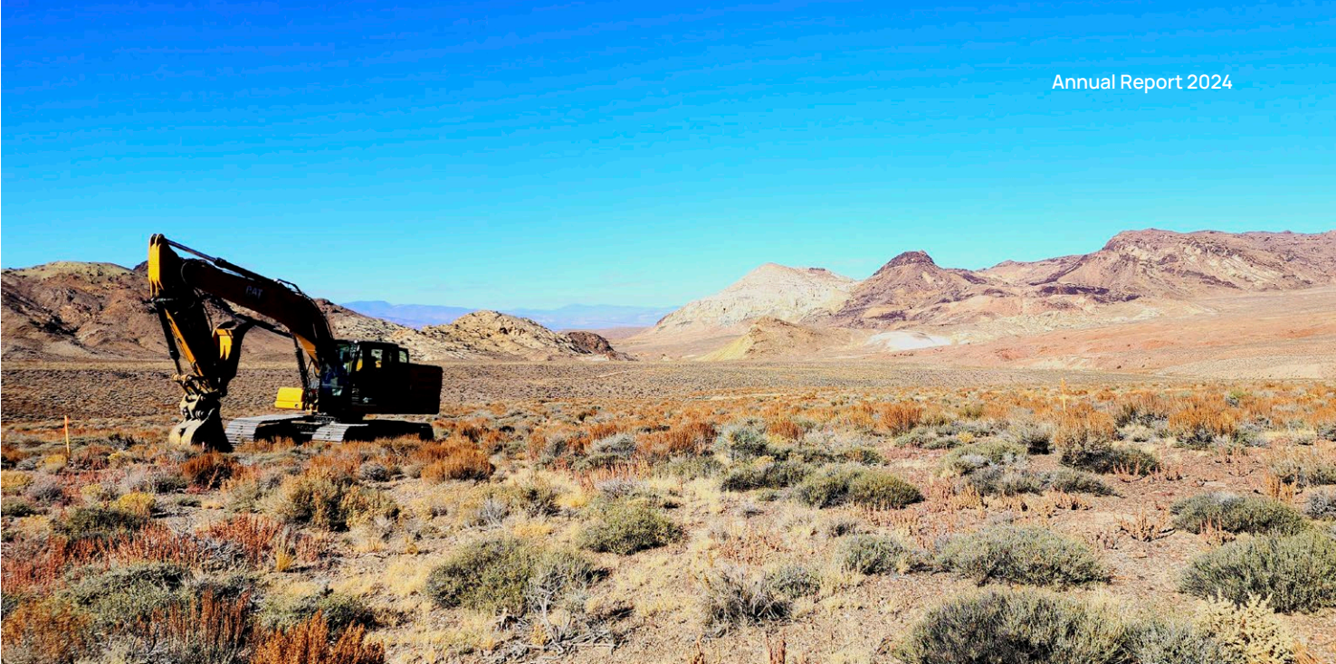
Drill pad preparation ahead of geotechnical drilling
