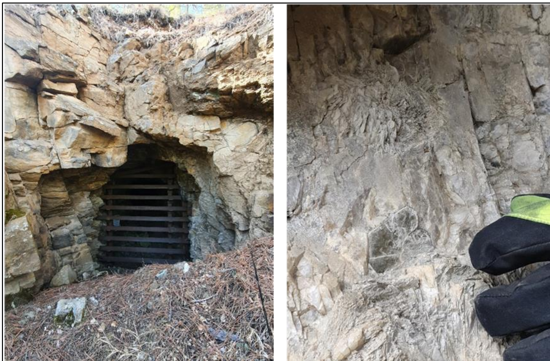
Figure 8: Tunnel entrance to the No. 9 Mine that contains a spodumene rich zonation.
