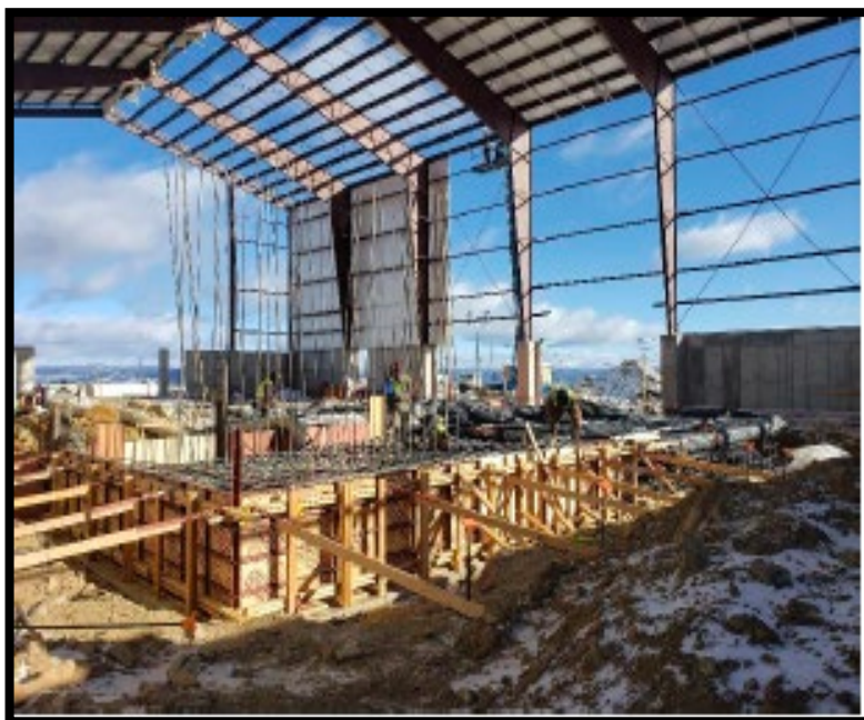
SAG and ball mill form work
