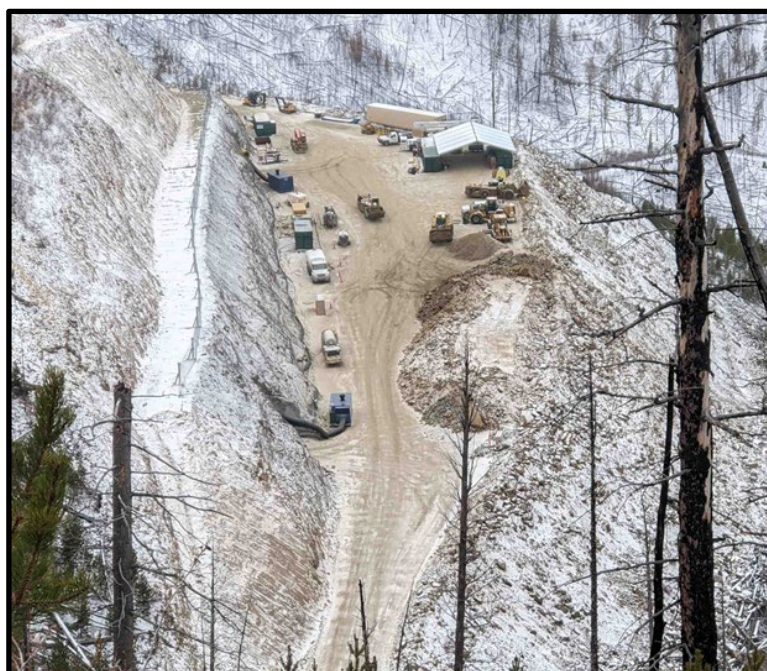
Portal bench infrastructure
