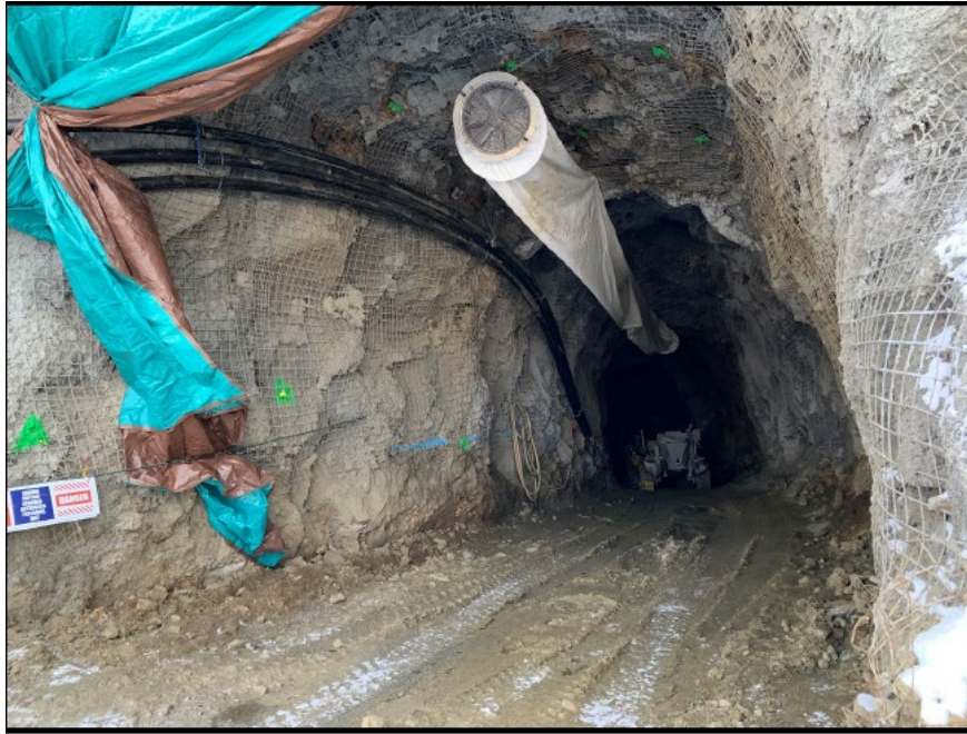
West Portal development with installed ventilation
