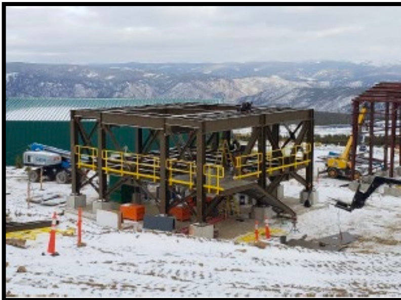
Fine ore bin and mill feed conveyor base structure
