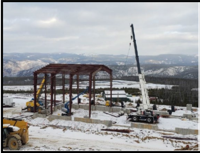
Flotation building progress
