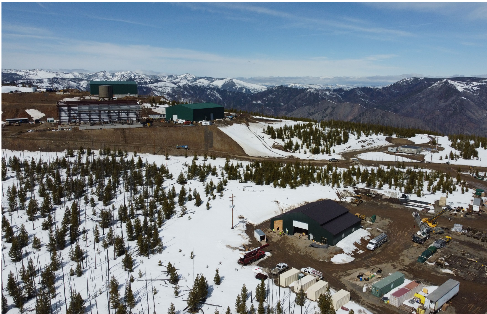
Surface Construction at ICO (March 2022)
