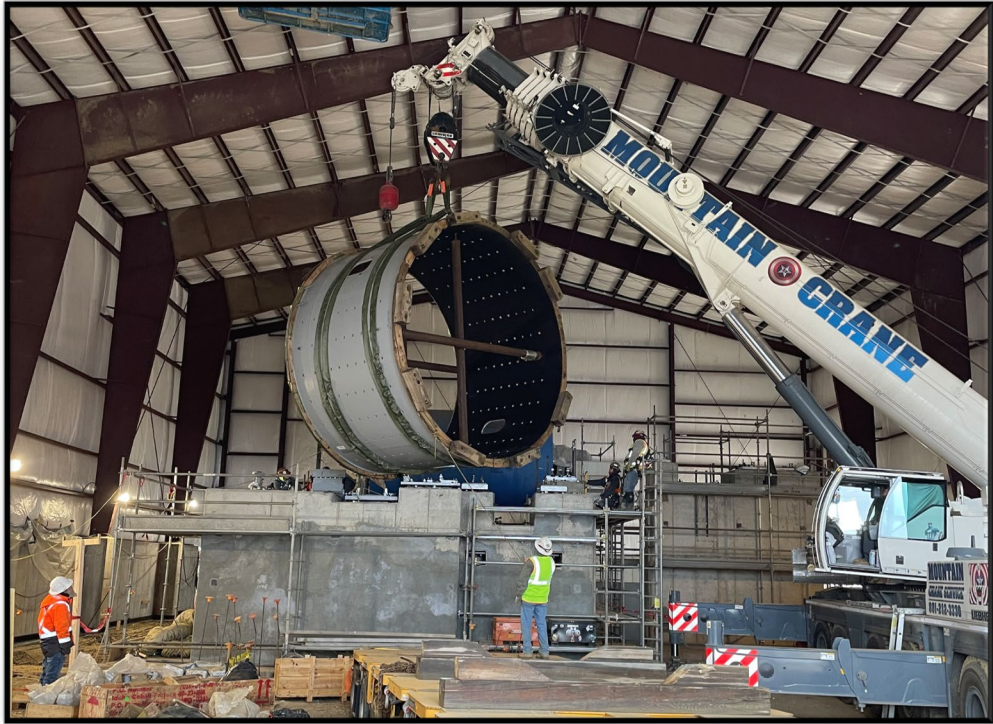
SAG Mill Shell Installation
