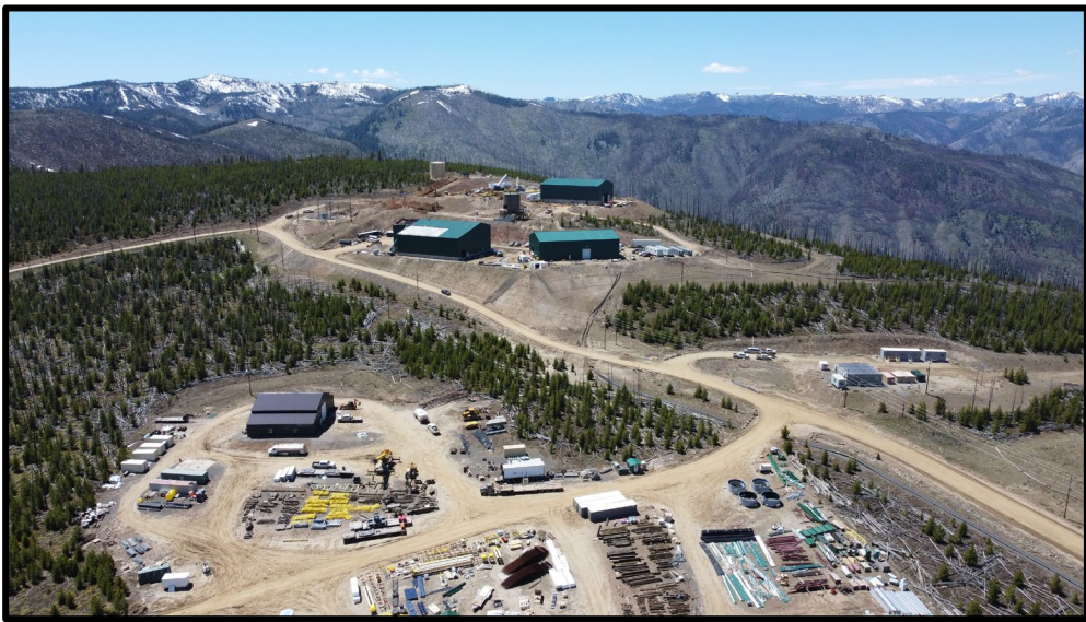
ICO Surface Facilities Progress
