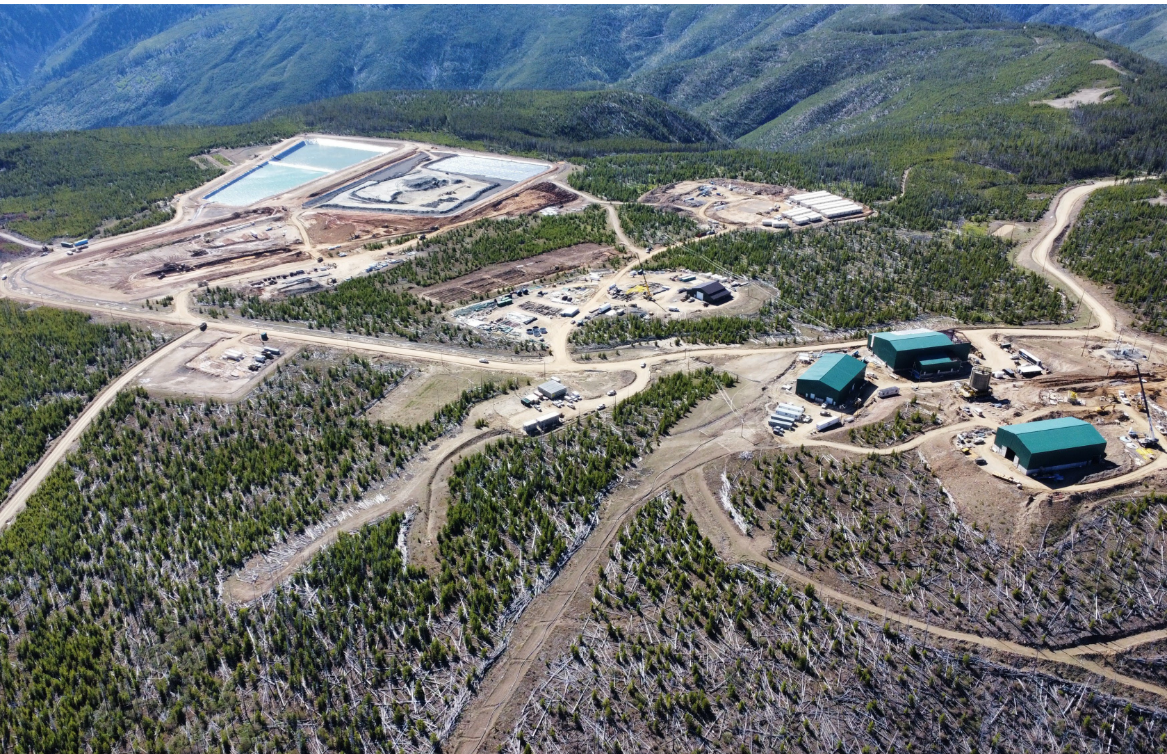
Surface construction at ICO (June 2022)
