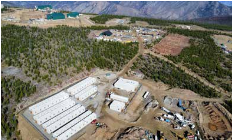
Accommodation camp (October 2022)
