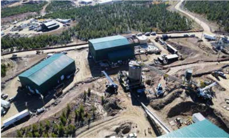
Surface construction (October 2022)
