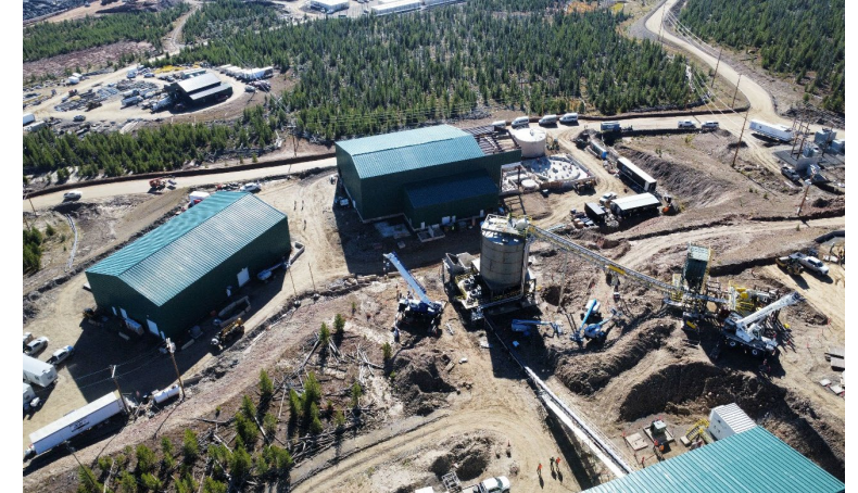
Surface construction (October 2022)
