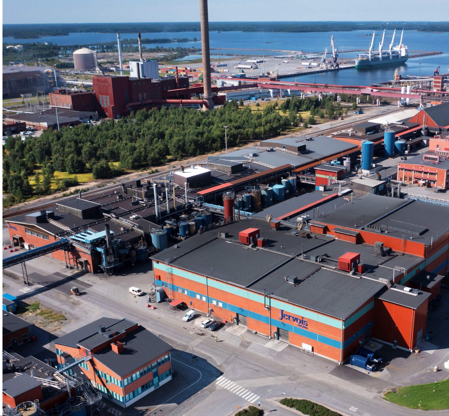
Kokkola manufacturing facility
