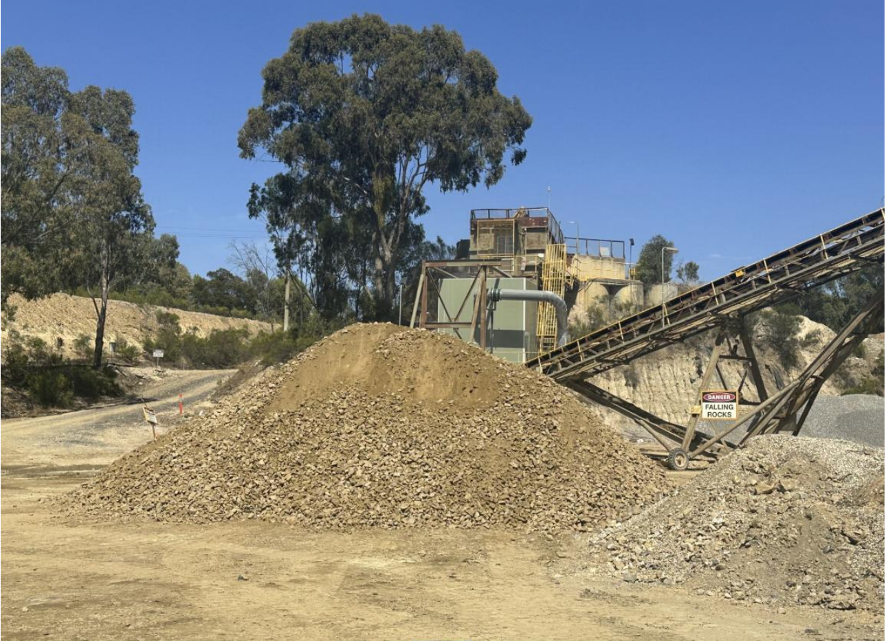
Figure 2, Union Hill Mullock material ready to be processed
