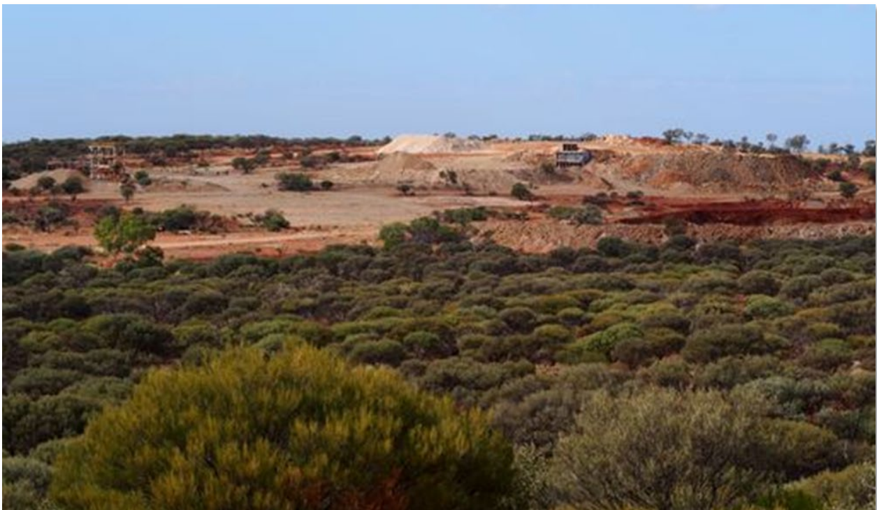
Figure 1: Looking south over area of major concentration of drilling (middle ground), showing pit bunding (centre right), with remnant ore and plant area shown (back ground).
