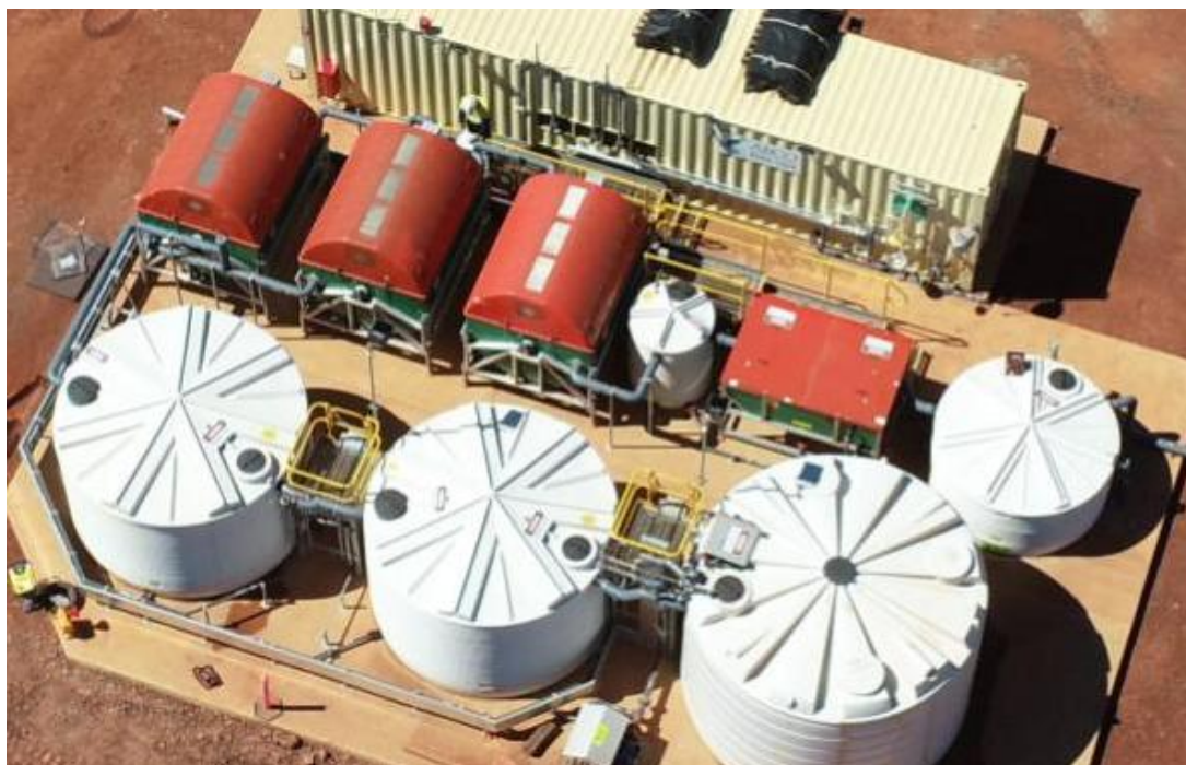
Figure 21: Example RBC type WWTP installed at Newmont Tanami Operations, NT (Ref: ABCO)
