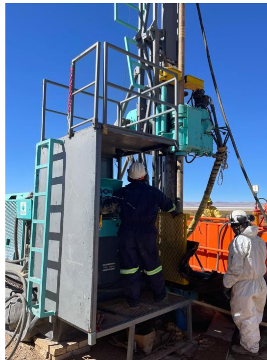
Figure 3: Drill rig operating on SOZDD001
