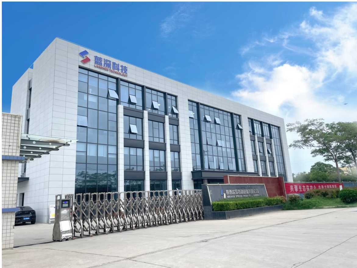
Figure 4: Lanshen Factory, Shaanxi Province, China
