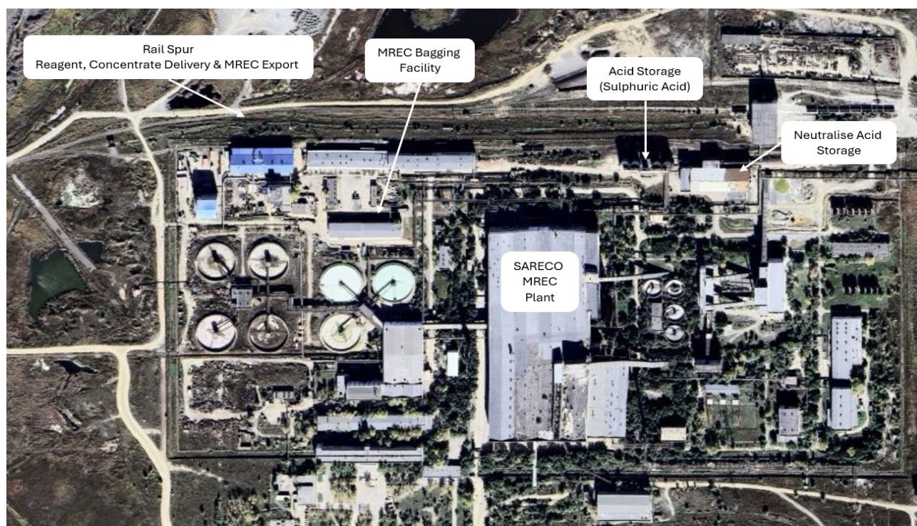
Picture 1. Site layout of the SARECO MREC Facility, highlighting key installed infrastructure including the main processing plant, sulphuric acid storage and neutralisation facilities, MREC bagging and dispatch area, and dedicated rail spur for reagent delivery, Concentrate receive and MREC export
