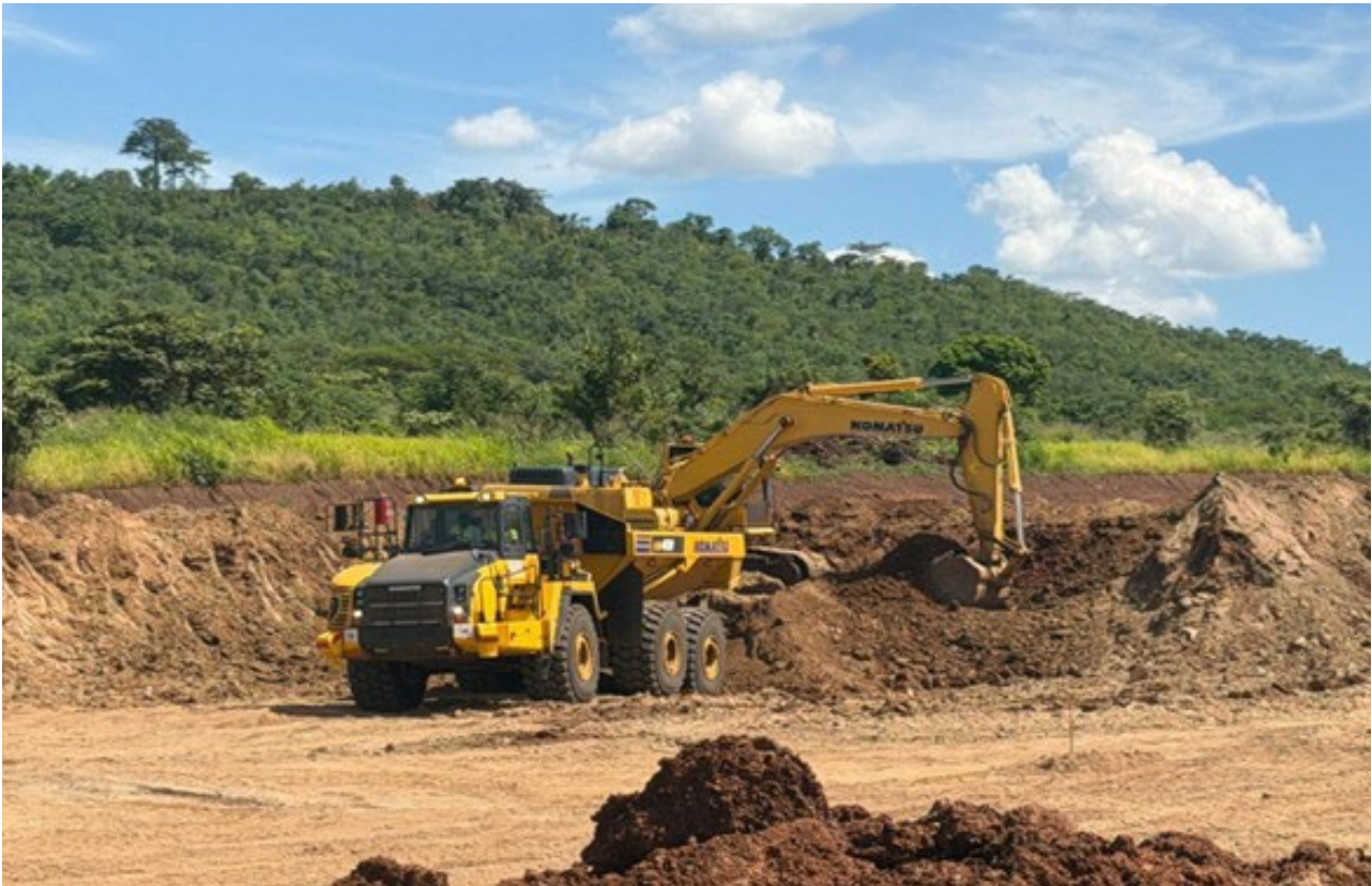
Picture 3. Owner-operated mining fleet executing TSF earthworks
