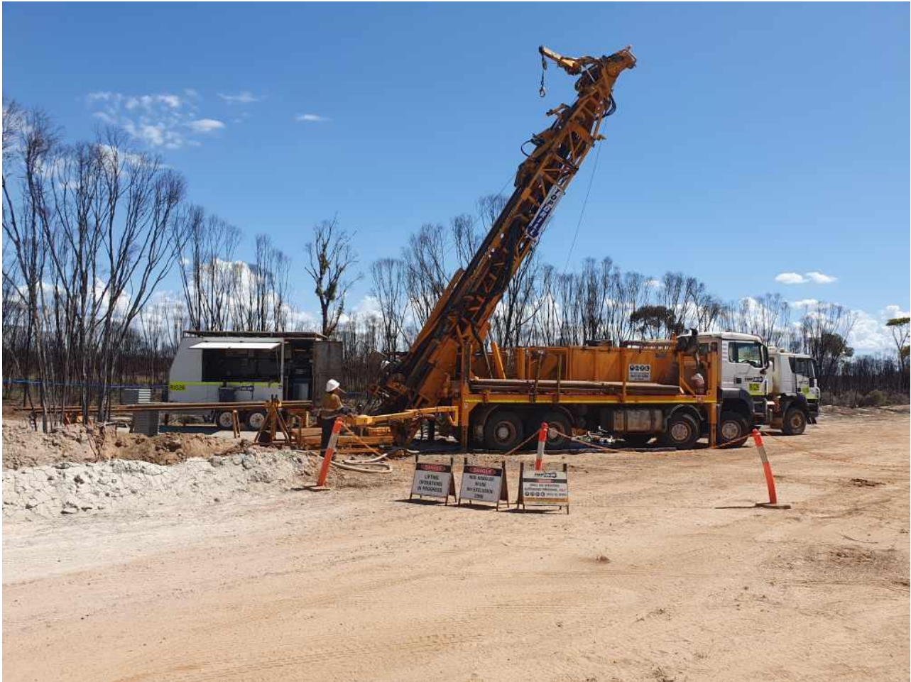
Figure 2 : Topdrill diamond drilling rig on site at Lady Grey Project Mt Holland
