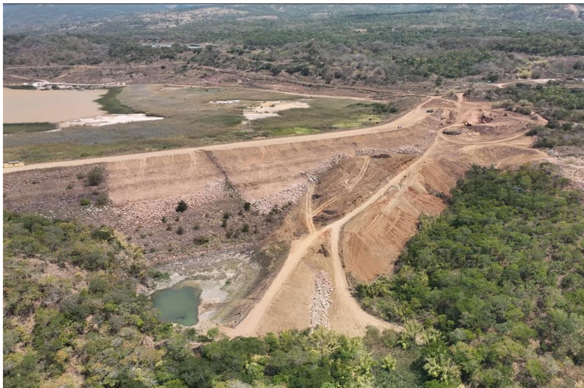
Figure 6: TSF lift works in progress
