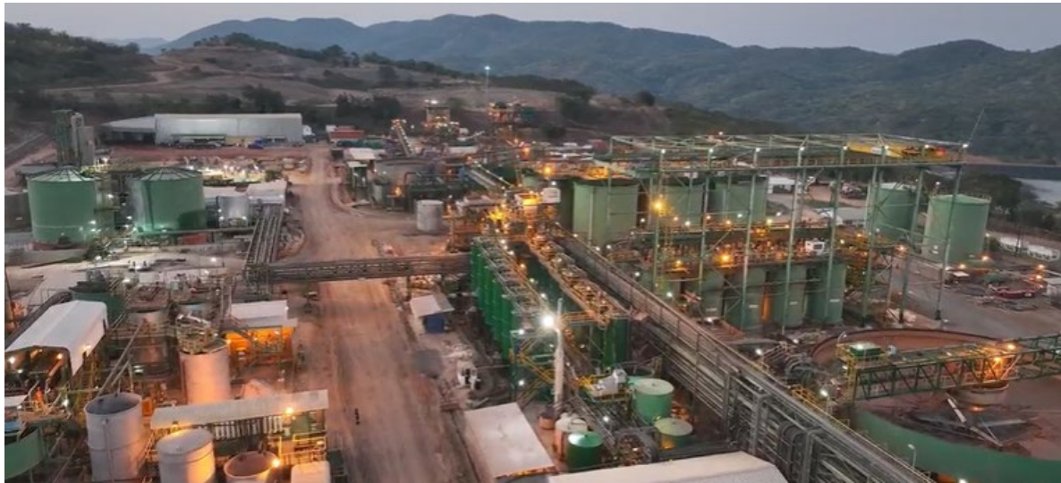
Figure 5: Leaching, RIP, elution and precipitation circuits
