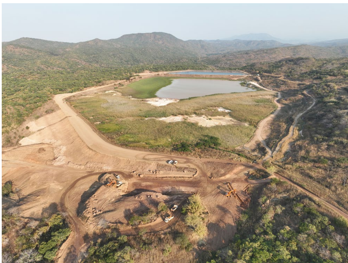
Figure 9: TSF lift works in progress
