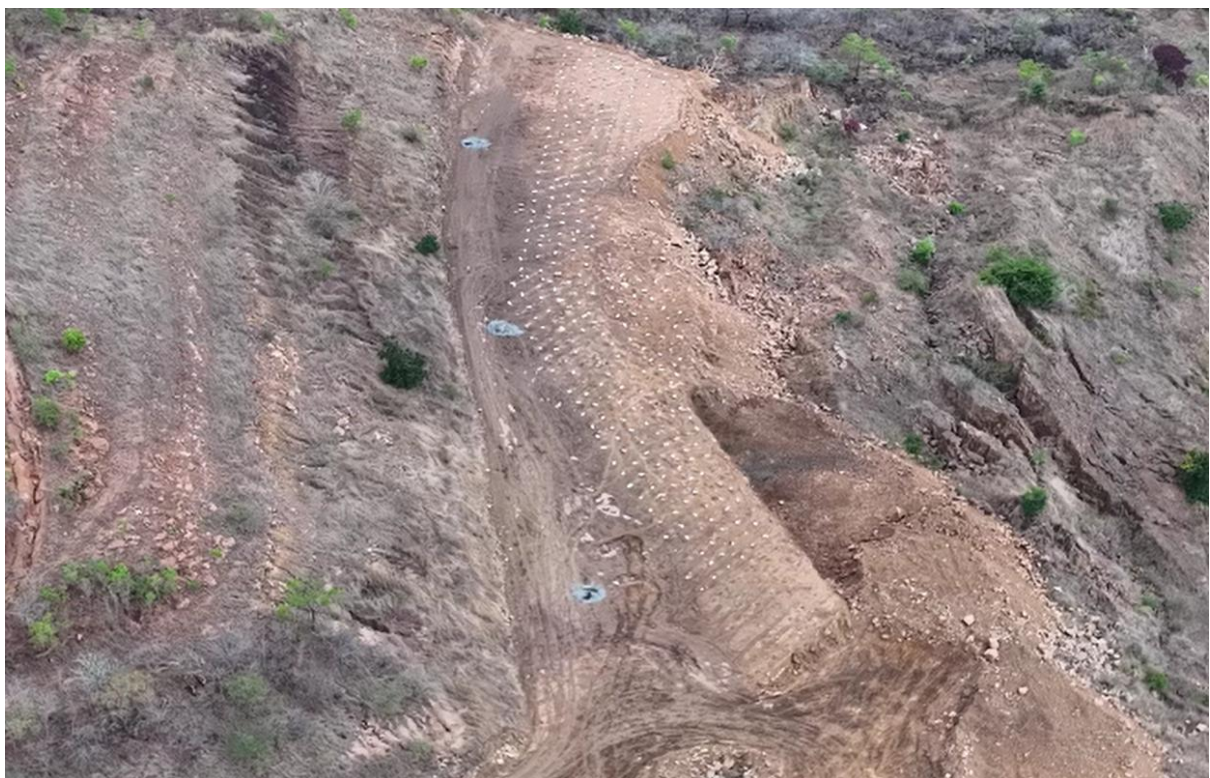
Figure 2: Aerial image of blast hole pattern for Kayelekera's open pit
