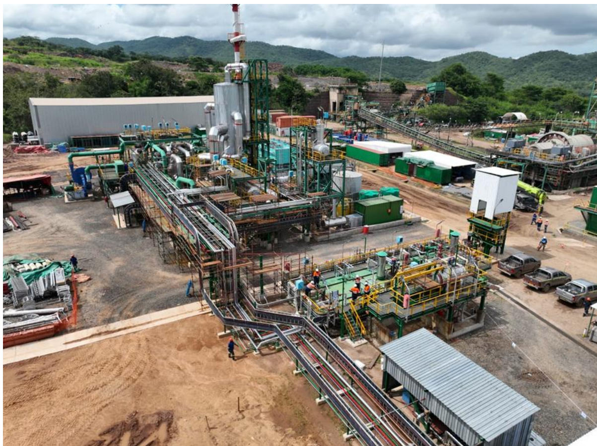
Figure 4: Acid plant (late March)
