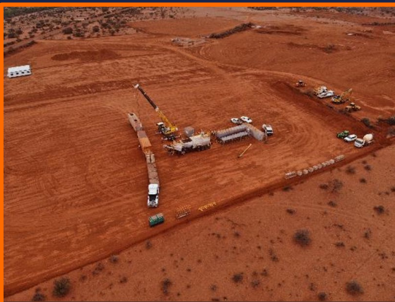
Concrete batch plant mobilised and operational
