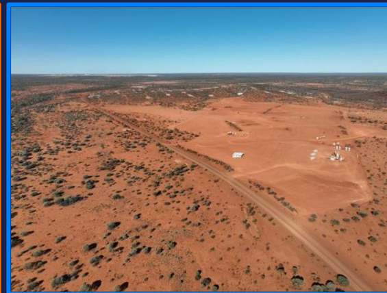
Plant site cleared
