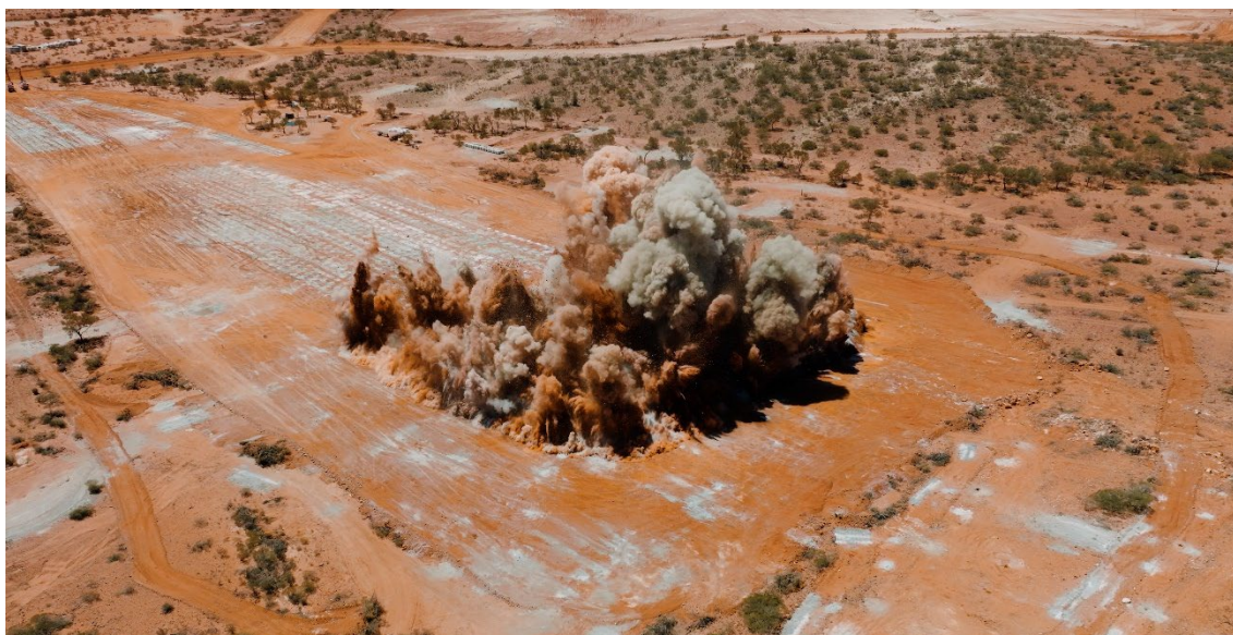
Figure 1: Aerial view of the first blast for the Mt Mann open pit
