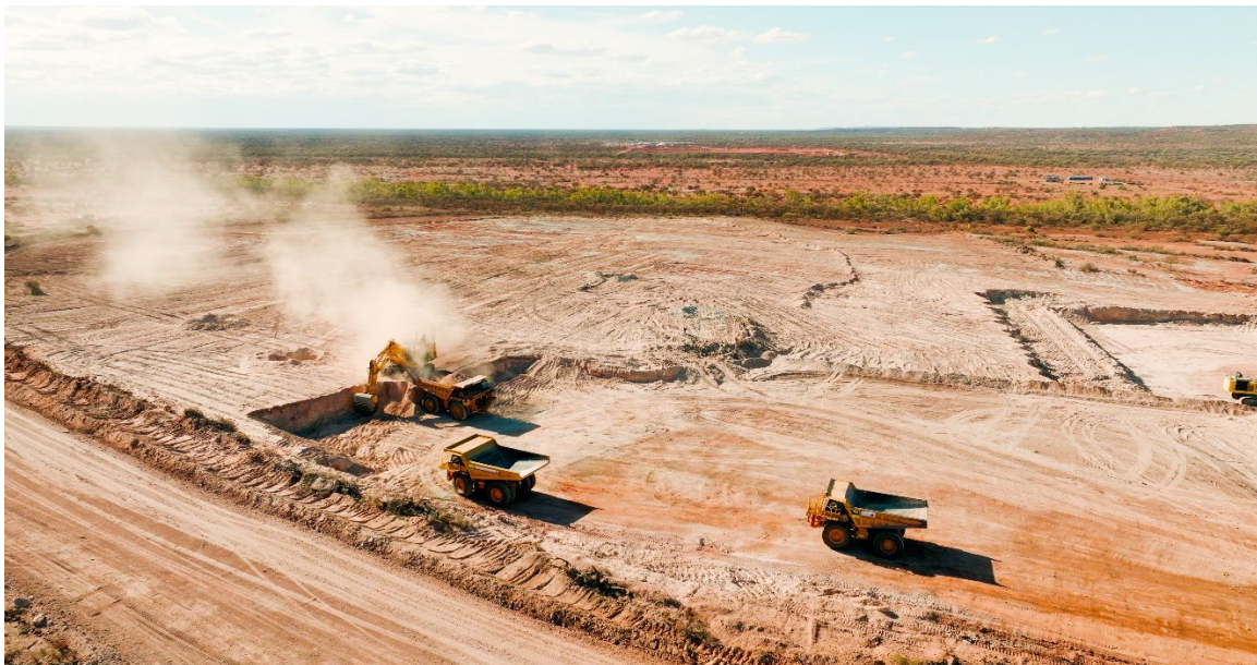
Figure 2: Load and haul operations underway in the Kathleen's Corner open pit
