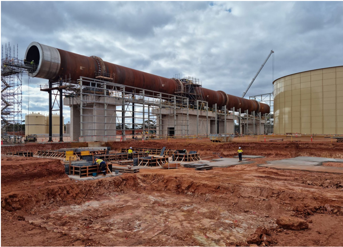
Waste Gas Plant foundation excavations and formwork progressing, with assembled kiln in background
