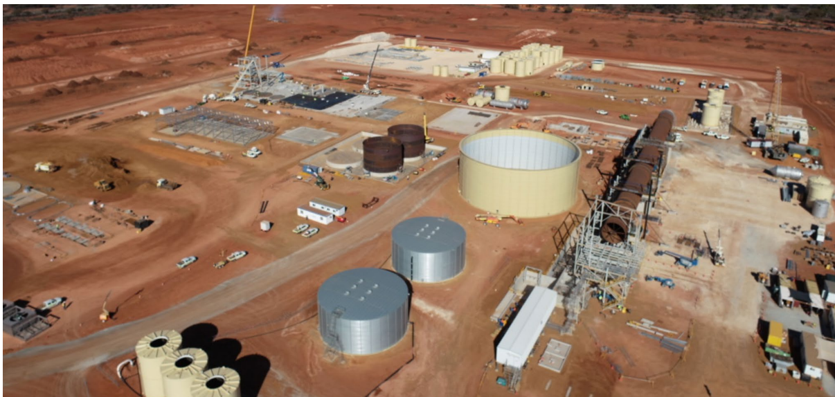
Aerial view of Kalgoorlie construction works, June 2022
