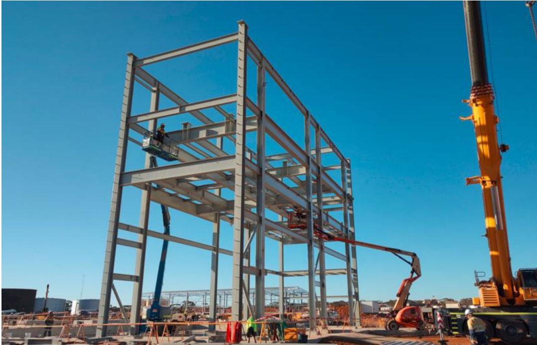
Filter building foundations complete, flooring complete for 30% of building and structural steel progressing
