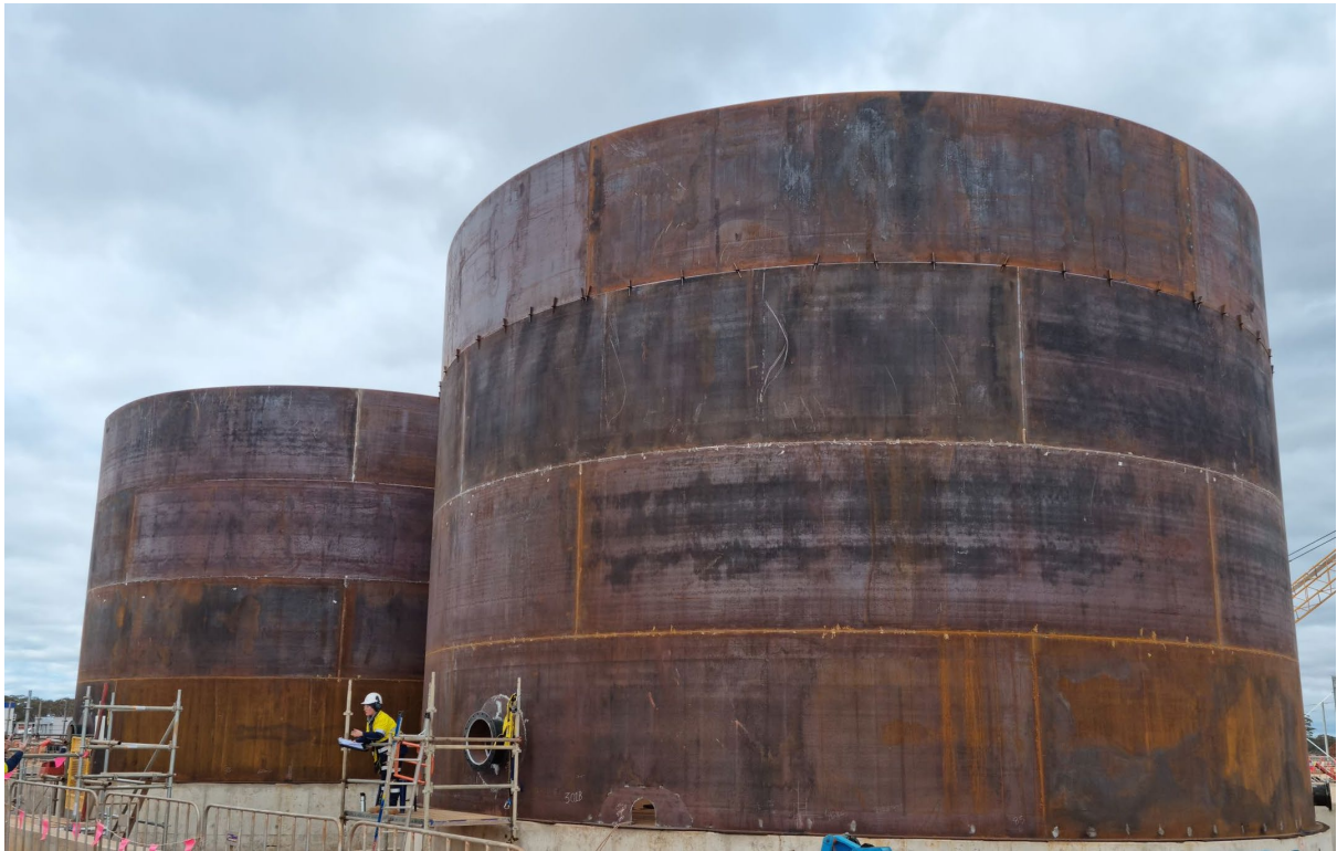
Fabrication of two 1300m 3 tanks complete
