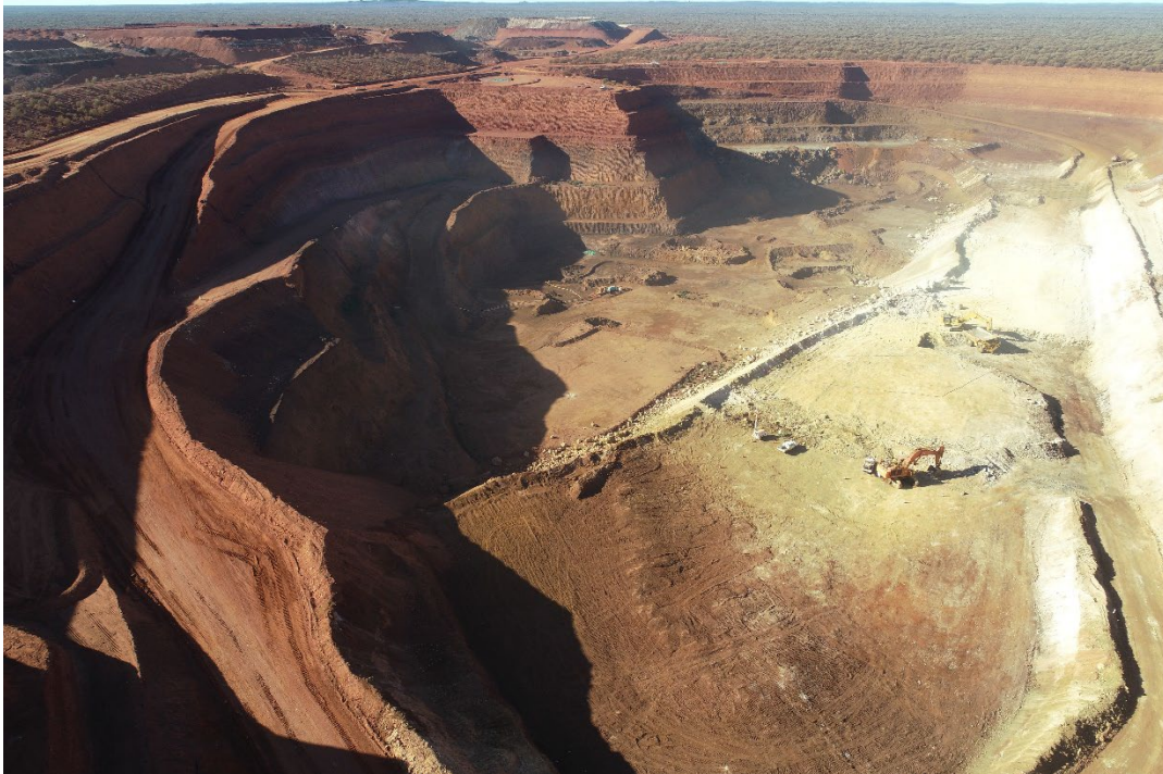
Photo: Mt Weld open cut mine as at 6 July 2022 showing Campaign 4 cutback on the right hand side
