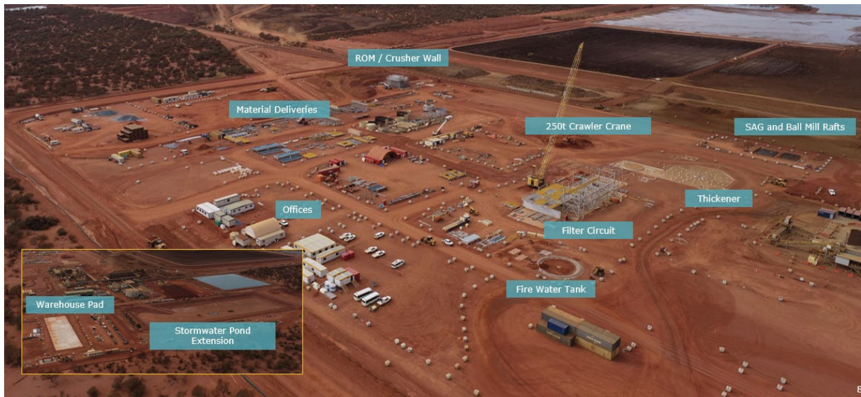
Mt Weld Expansion - Site Construction General Overview
