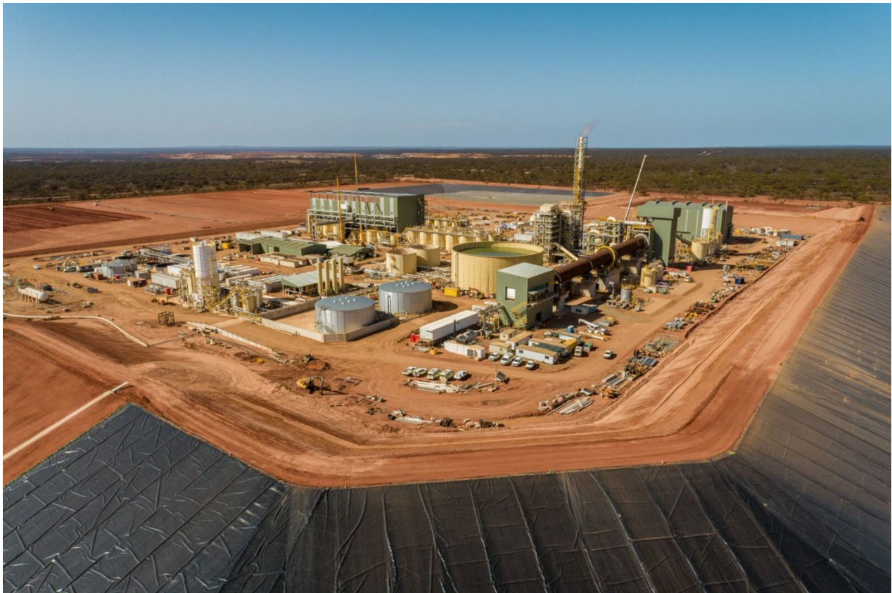
Lynas Kalgoorlie Rare Earths Processing Facility
