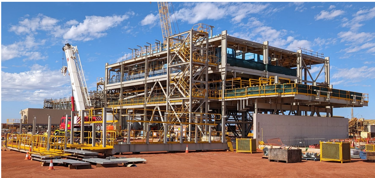
Mt Weld Expansion – Stage 1 (Thickener and Filter Circuit)
