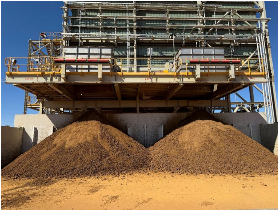
Concentrate Dewatering Circuit in Production
