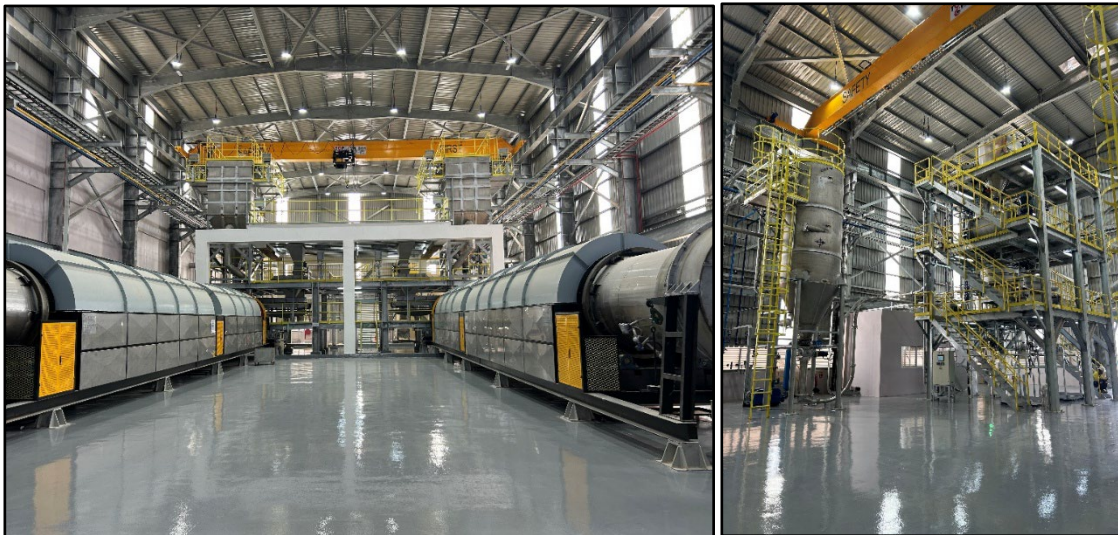
Photo: New furnaces for calcination
