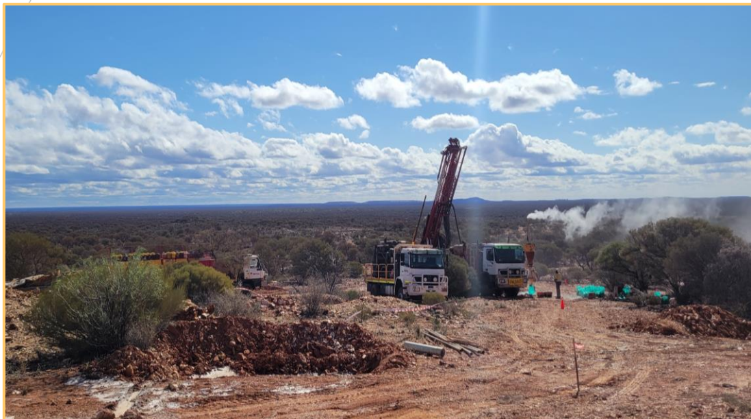
Figure 1 RC rig drilling at the Golden Crown Prospect, looking west, Sons of Gwalia mullock dumps centre background behind rig
