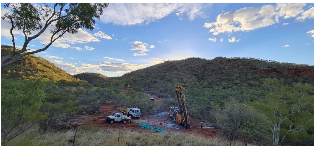
Figure 1: MI21RC07 drill setup nearing completion of 2021 drill program
