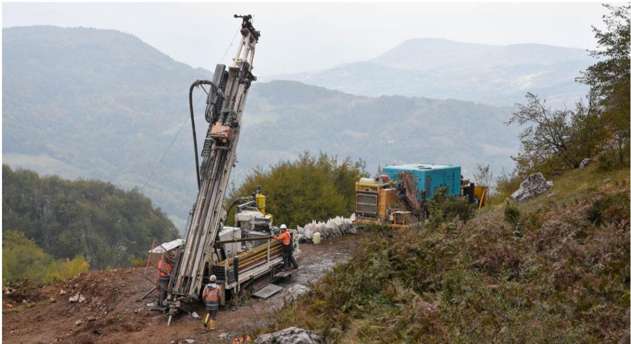
Figure 1: Drilling in the Bobija mine area.
