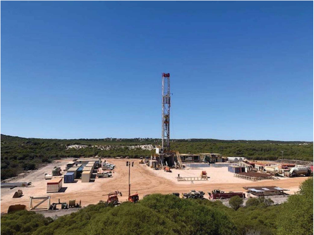
Figure 3: Ensign 970 drilling at Cervantes-1 location
