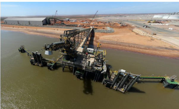
Transhipping wharf installation completed
