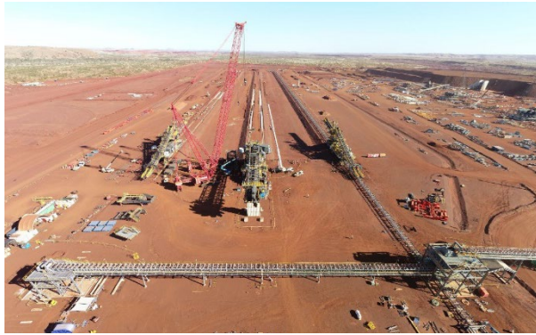
Stacker and reclaimer assembly ongoing
