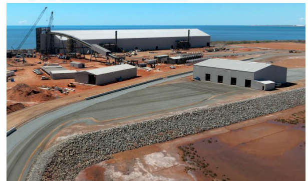
Product storage facilities at Port of Ashburton
