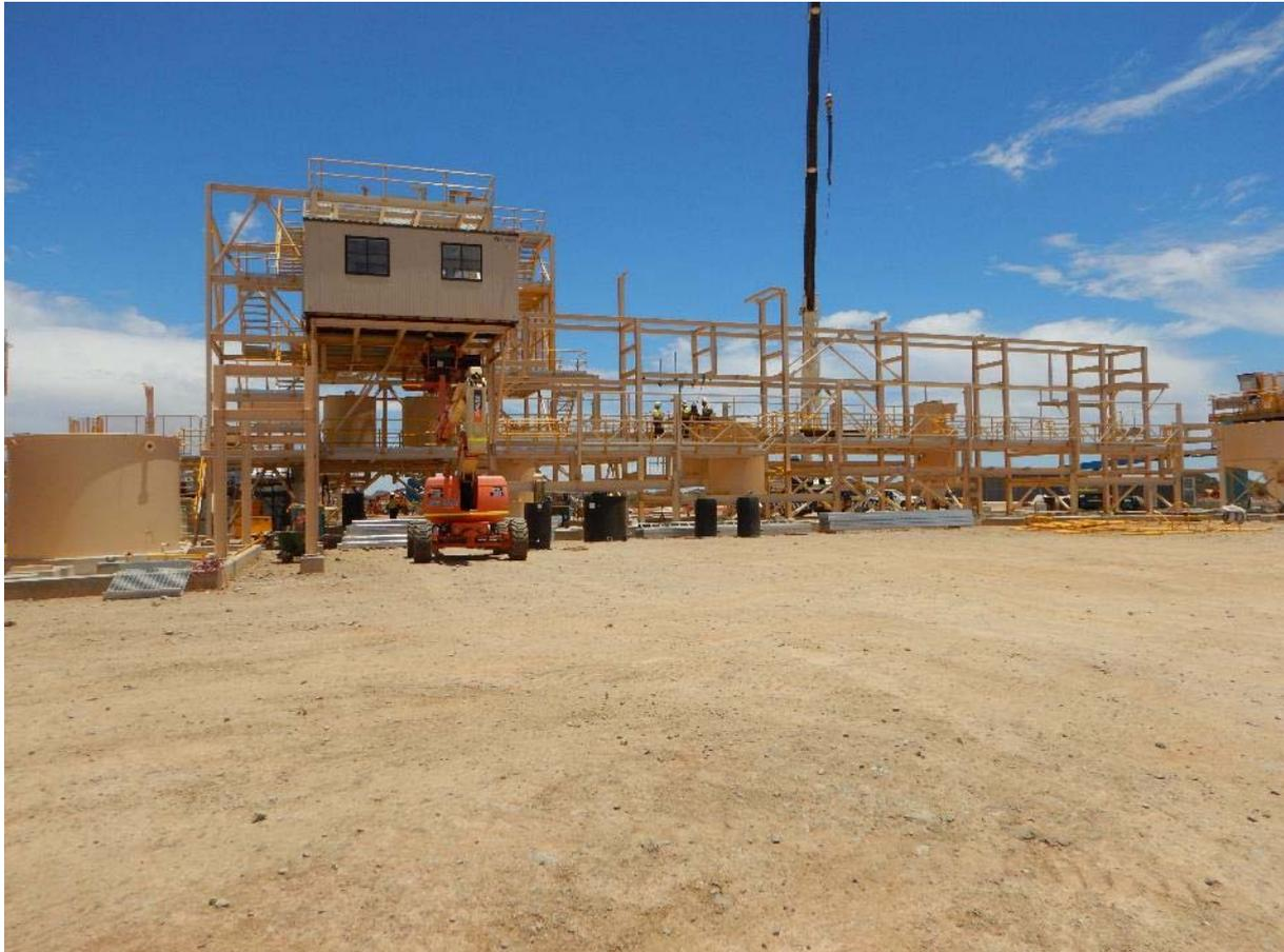
**Figure 6.** Mill control room installed with flotation circuit steelwork underway.
