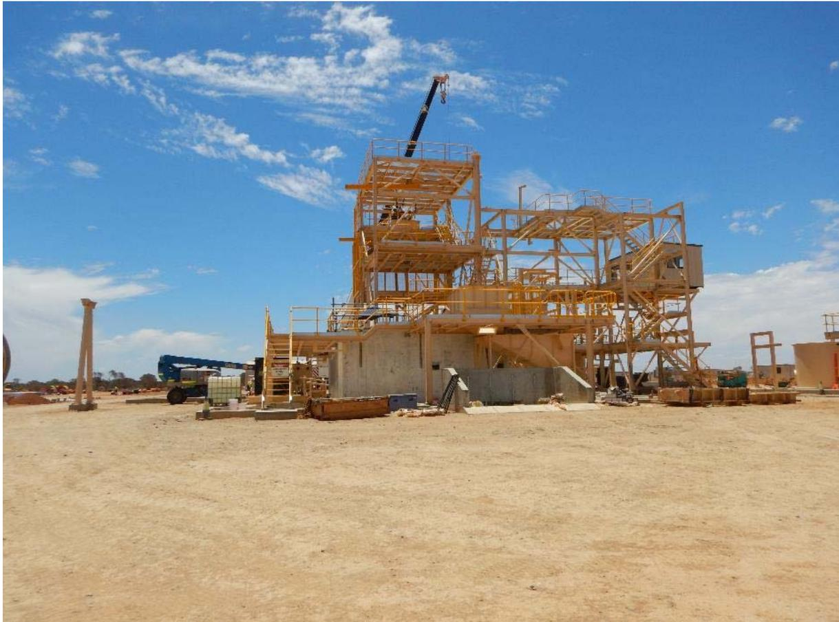
**Figure 4.** Mill plinth with gravity circuit tower and mill control room installed.
