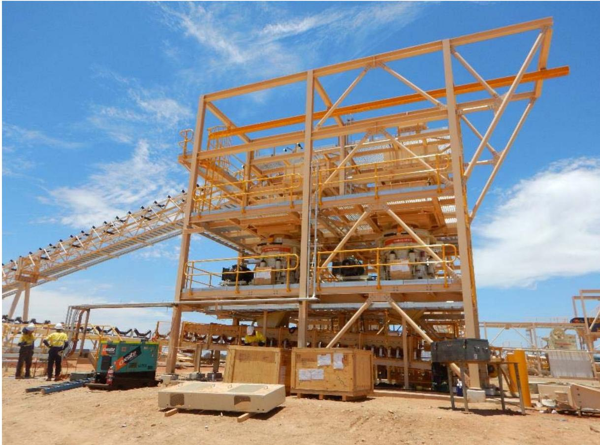
**Figure 2.** Crushing tower with secondary and tertiary crushers installed.
