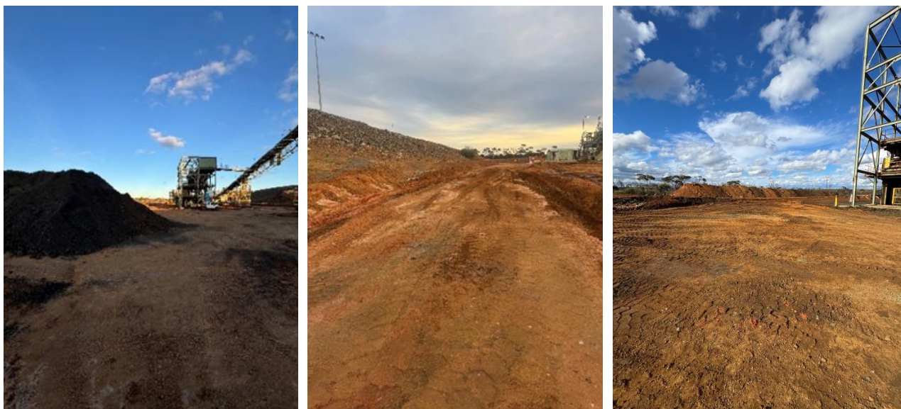
Figure 3: Boxing out of CBC footings ahead of commencement of site civils
