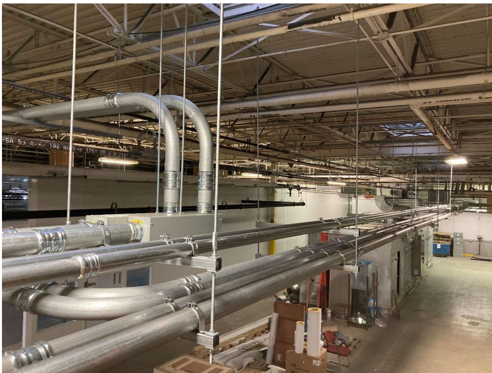
Figure 4: Low Bay electrical conduit installation
