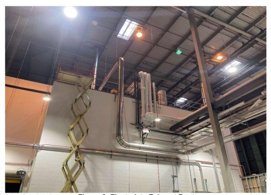
Figure 2: Electrolyte Exhaust Duct
