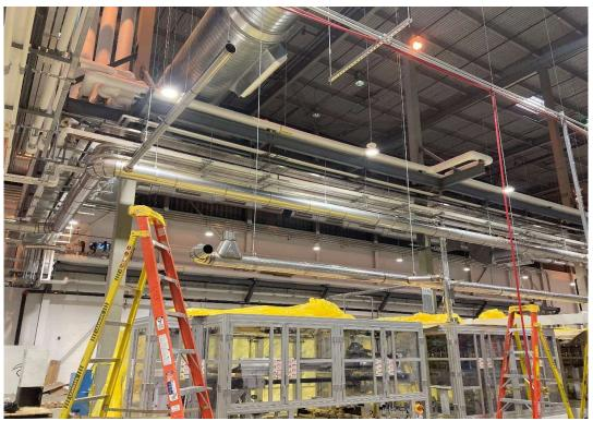
Figure 1: Degassing Ductwork
