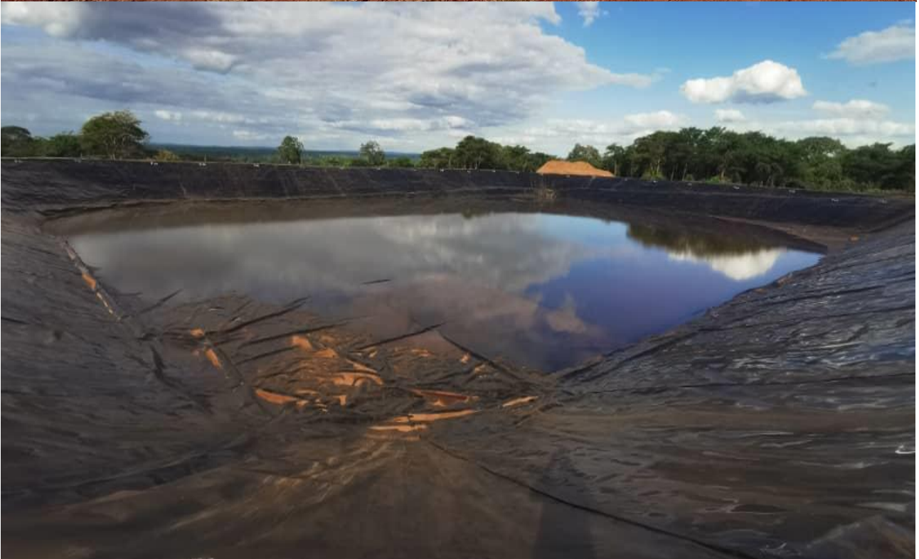
Figures 3 and 4: Nachu Water Storage Dam
