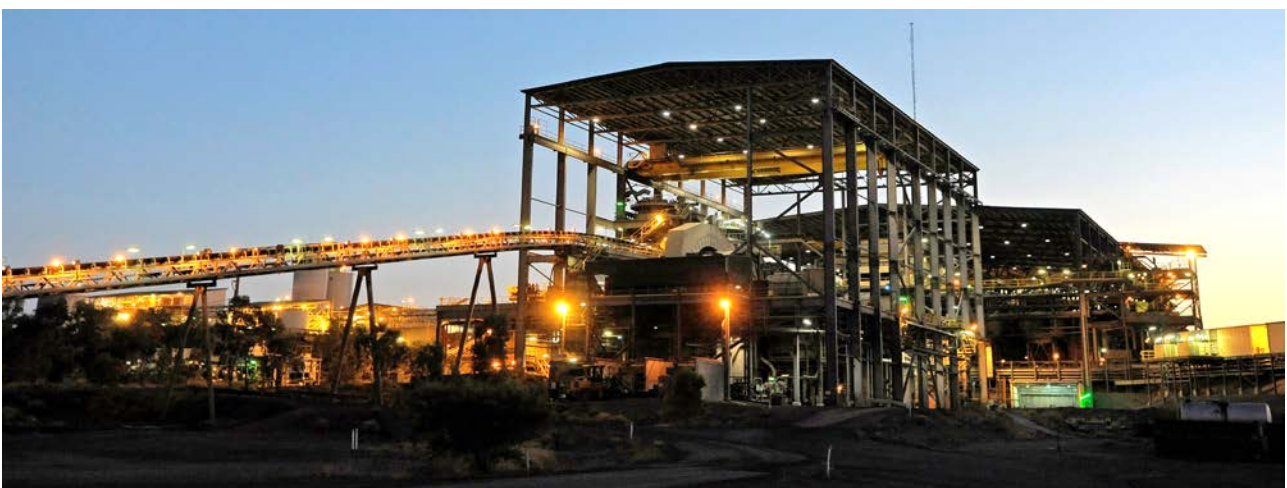
Figure 1: New Century's 7Mtpa Processing Plant to be used to restart processing at the Century Zinc Mine
