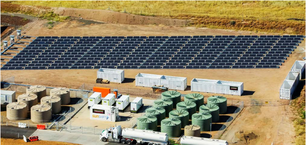
Figure 13: Modular solar system to be installed at the Century Mine
