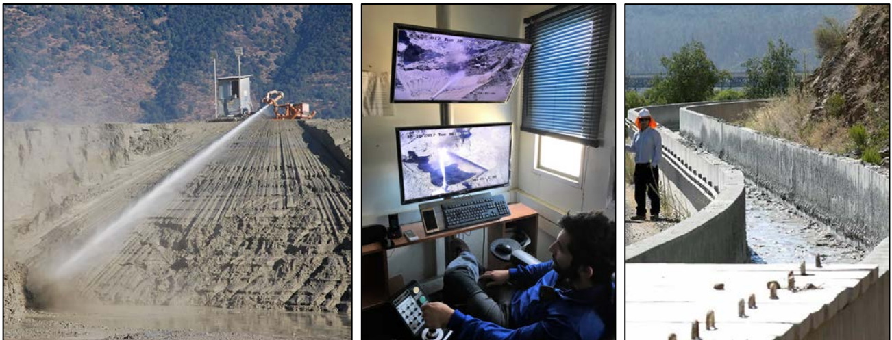
Figure 4: MVC hydraulic mining operations and fresh tailings transportation infrastructure (67Mtpa)
