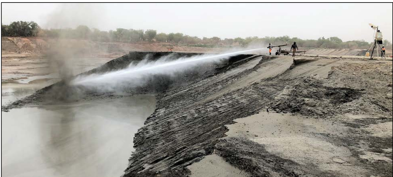
Figure 1: Paragon undertaking hydraulic mining operations at Randgold's Morlia Mine, Mali (15Mtpa)
