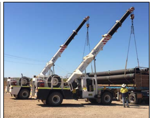
Figures 13 & 14: Delivery of offsite fabricated tailings HDPE pipework and feed preparation equipment during the month of June
