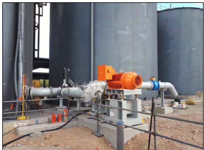
Figures 7 & 8: Piping reconfiguration activities within the Century Processing Plant for tailings reprocessing (left) and tailings ore Feed Transfer Pump installation (right)
