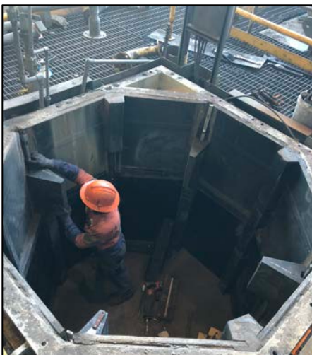
Figures 11 & 12: Relining and refurbishment of the Vertical Fine Grind Mills (left) and fusion welding of the tailings ore Feed Pipeline into the Century Processing Plant (right)
