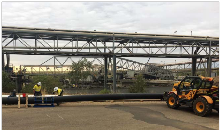
Figures 11 & 12: Relining and refurbishment of the Vertical Fine Grind Mills (left) and fusion welding of the tailings ore Feed Pipeline into the Century Processing Plant (right)
