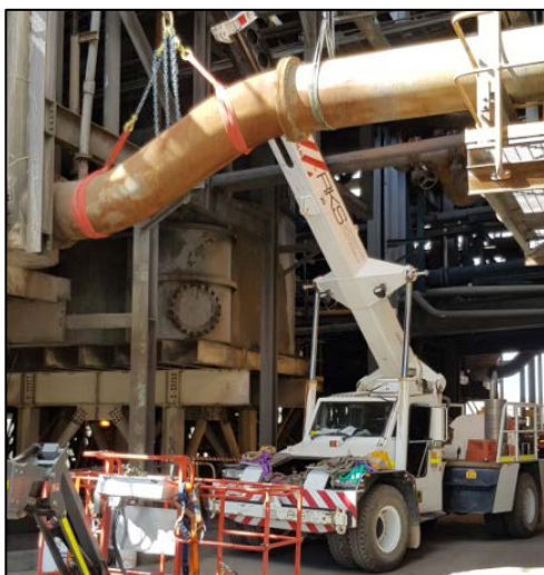
Figures 7 & 8: Piping reconfiguration activities within the Century Processing Plant for tailings reprocessing (left) and tailings ore Feed Transfer Pump installation (right)
