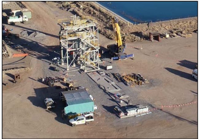
Figures 9 & 10: Tailings Feed Preparation area design overlaid on full site 3D lidar survey (left) and installation of the equipment ahead of commissioning activities (right)
