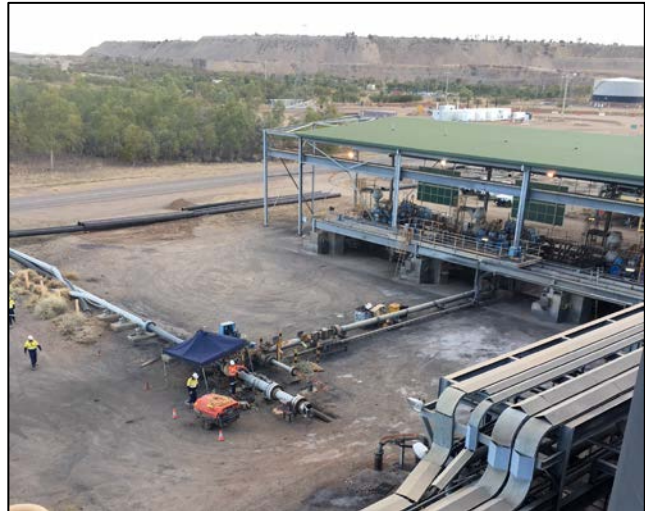
Figures 15 & 16: Rehabilitated area of the Slurry Pipeline previously excavated for cleaning pig removal (left) & New Century & Ausenco team members filling the Pipeline as part of water commissioning (right)
