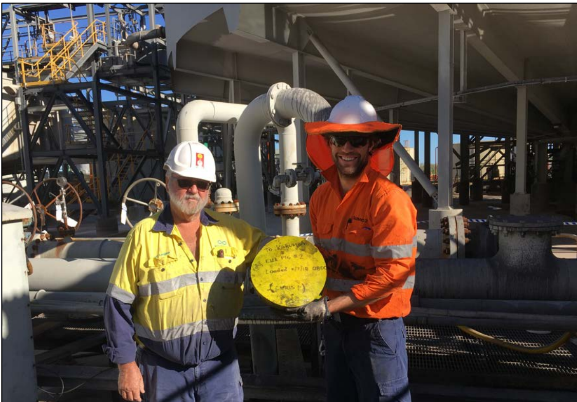
Figure 1: New Century Operational Support Officer Jeff Langton (left) and Ausenco Project Engineer Christian Small (right) with the second cleaning pig used to successfully commission the Concentrate Slurry Pipeline
