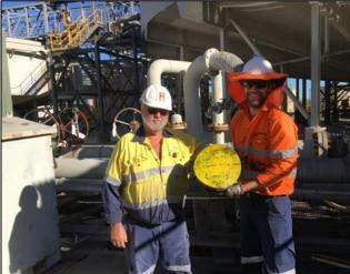
Figures 14 & 15: Loading of the cleaning pigs into the Concentrate Slurry Pipeline at the Lawn Hill Mine site (left)
