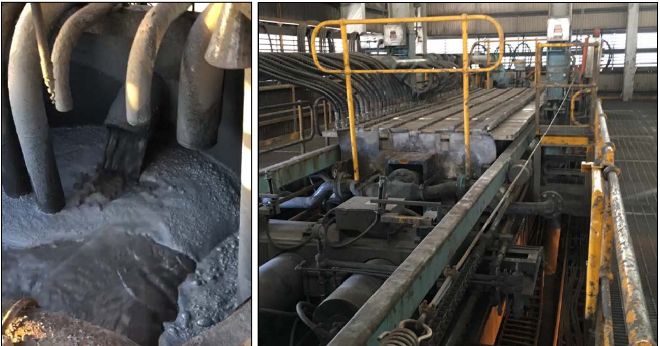
Figures 2 & 3: Zinc concentrate slurry entering the concentrate thickener from the slurry pipeline (left) and through one of the five filter presses (right) at the Karumba Port Facility
