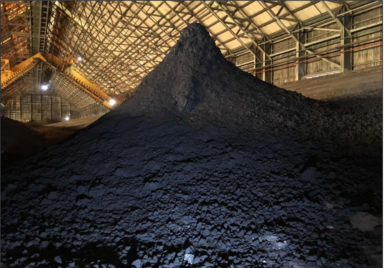
Figure 6: Initiation of stockpiling of zinc concentrate from the filter press facility into the Company's 80,000t capacity storage shed. Concentrate is removed for export from the storage shed via the mechanical reclaimer (located in the background of Figure 6) and loaded via conveyers directly onto the Company's transhipment vessel, the MV Wunma.
