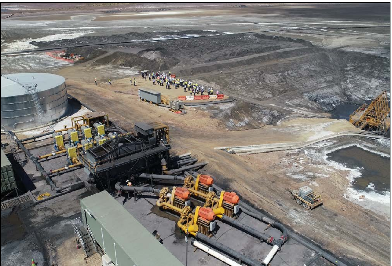
Figure 5: View of the hydraulic mining operations centre during the official reopening ceremony of the Century Zinc Mine on 14 September 2018
